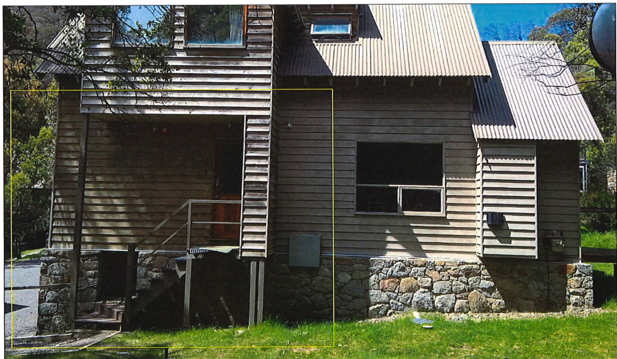
Figure 2: Area of works on northern elevation (Source: Department site inspection)
